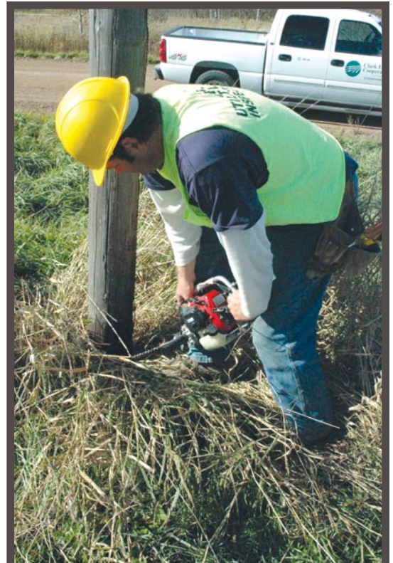
The next step is the bore testing of the pole if indicated. Above: Three bore holes are drilled into the pole to determine if the core of the pole is good and if other problems with the pole exist. Below: Special treated plugs are used to fill the holes left by the boring process. They are hammered in so they are secure.
